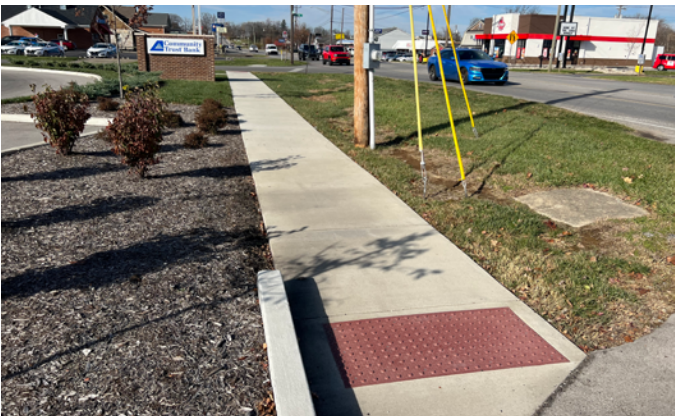
New sidewalk along south side, looking west
