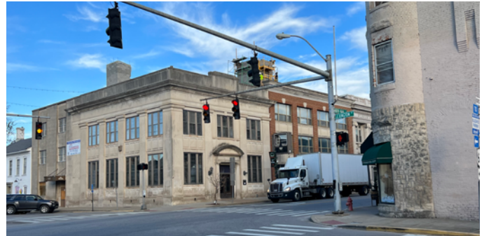
Main Street mast arm signalization
