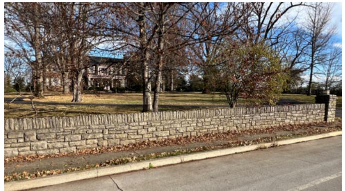
Existing stone masonry wall
