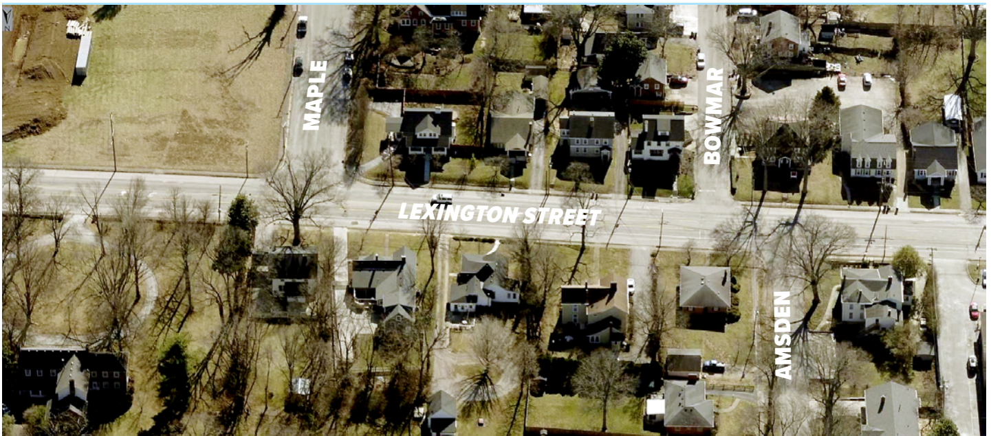
Segment 2B aerial, looking south
