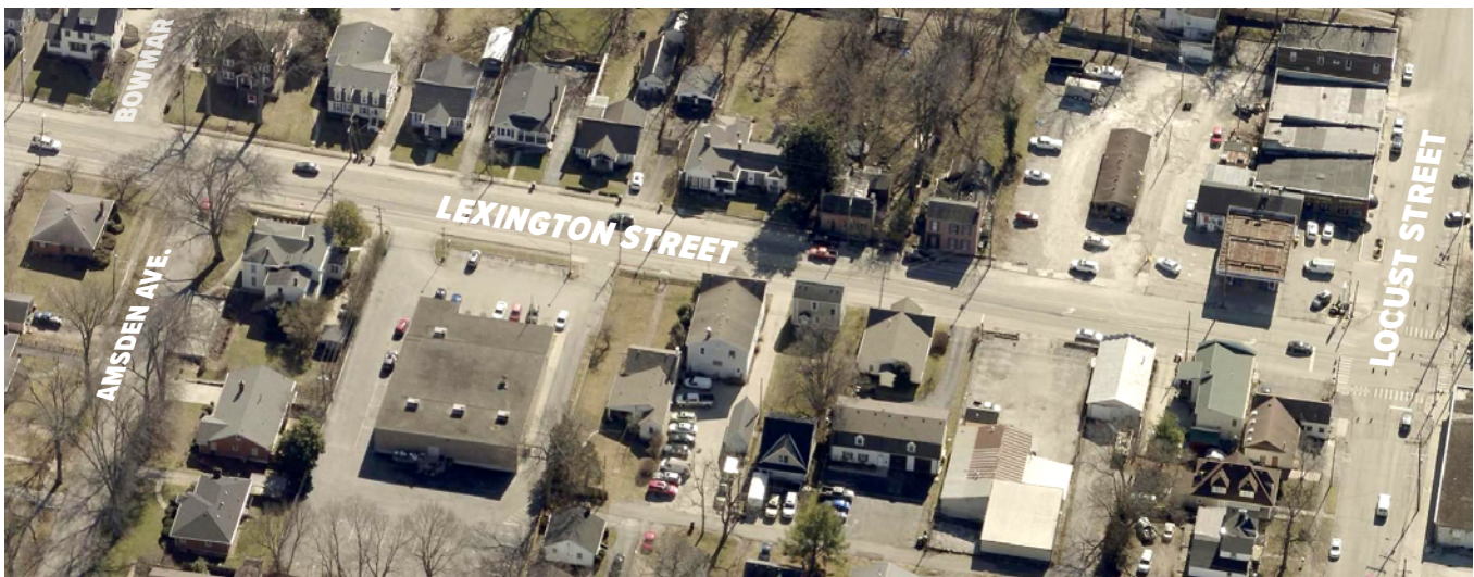
Segment 2A aerial, looking south
