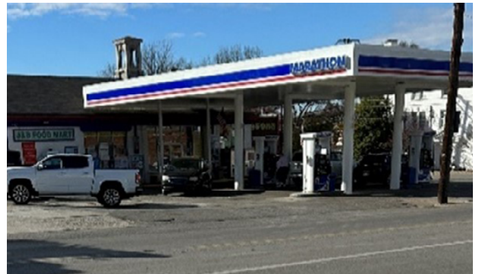
Potential HAZMAT Concern
